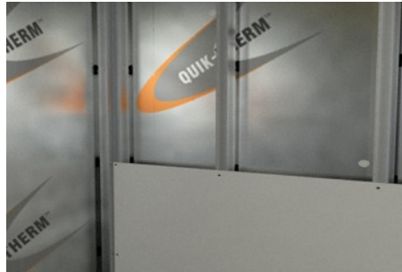
Interior Concrete Insulation System (CIS)
